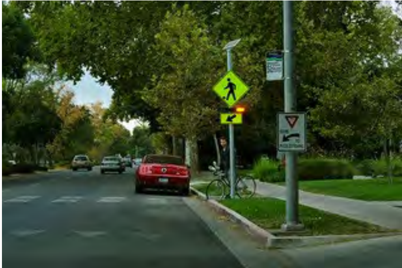
Rectangular Rapid Flashing Beacon (RRFB)
