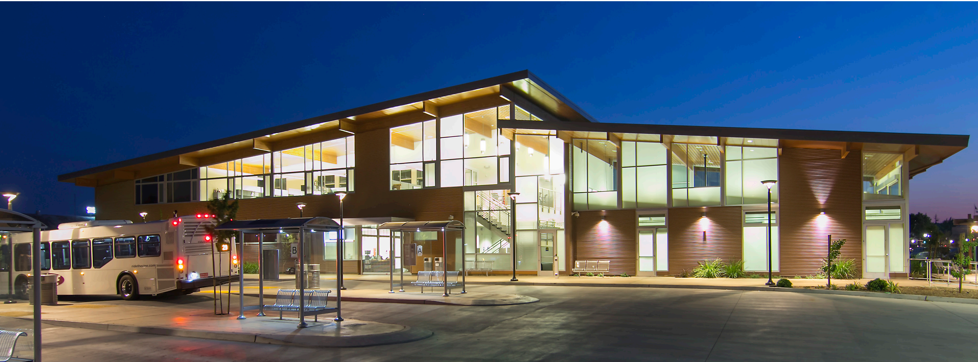
SOSCOL GATEWAY TRANSIT CENTER
