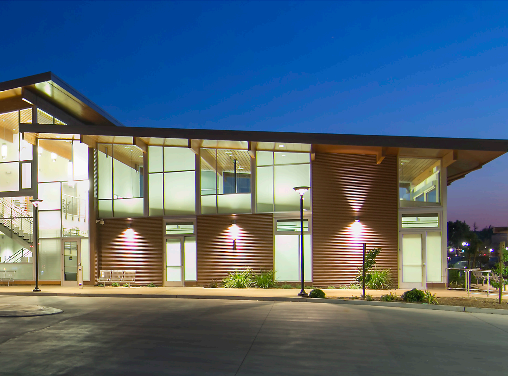
SOSCOL GATEWAY TRANSIT CENTER
