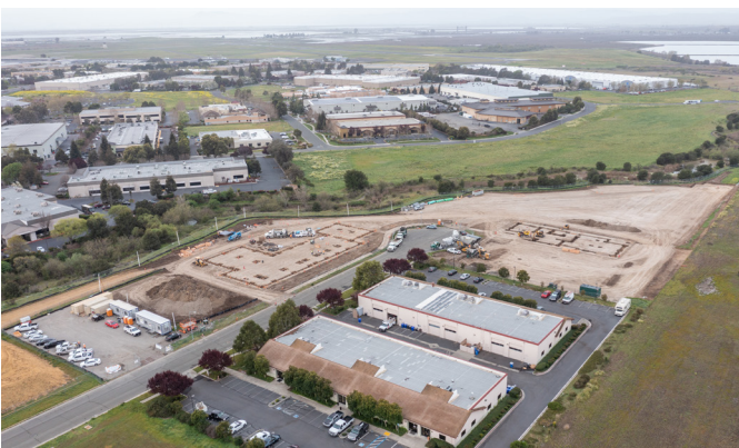
Current construction (March 2022)
