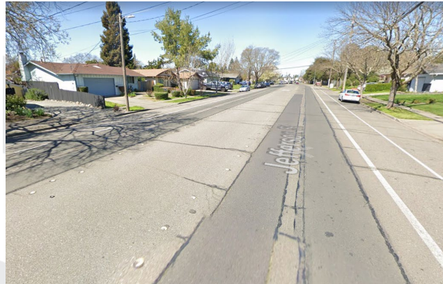
JEFFERSON STREET REHABILITATION
