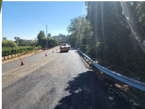
Repairs @ OSR & CVR
