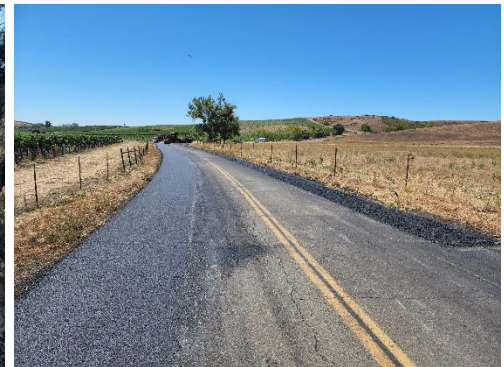
Repairs Buhman Ave.
