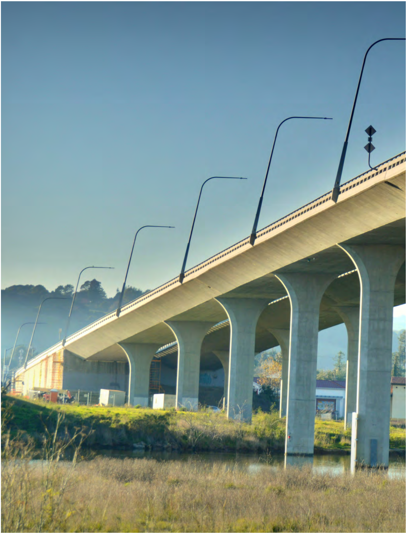
State Route 121 Maxwell Bridge over the Napa River
