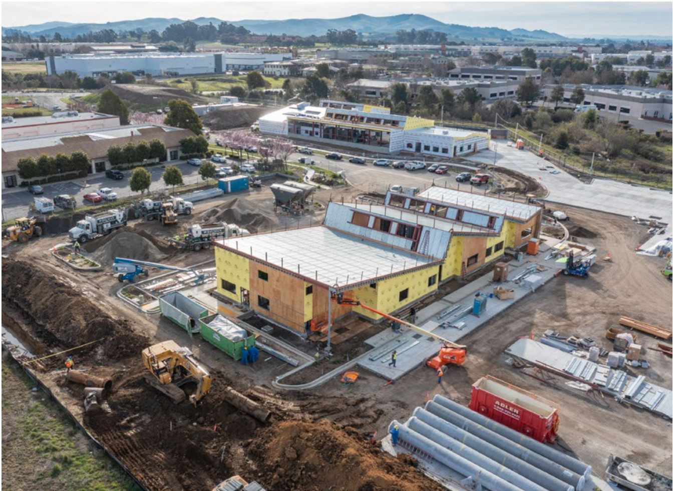
Current Construction, February 2023
