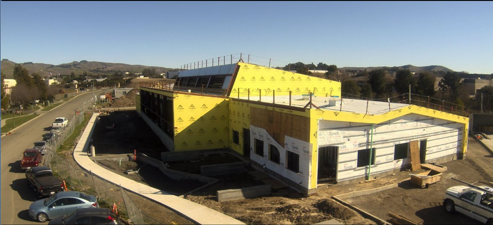
Vine Bus Maintenance Facility, February 2023
