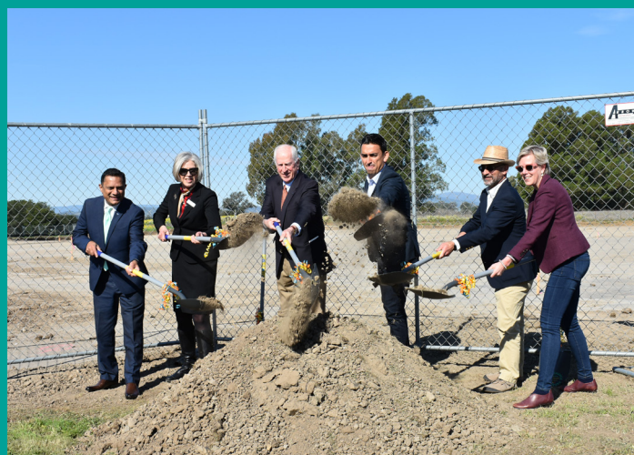
Transportation leaders break ground on the Vine Transit Bus Maintenance Facility.
