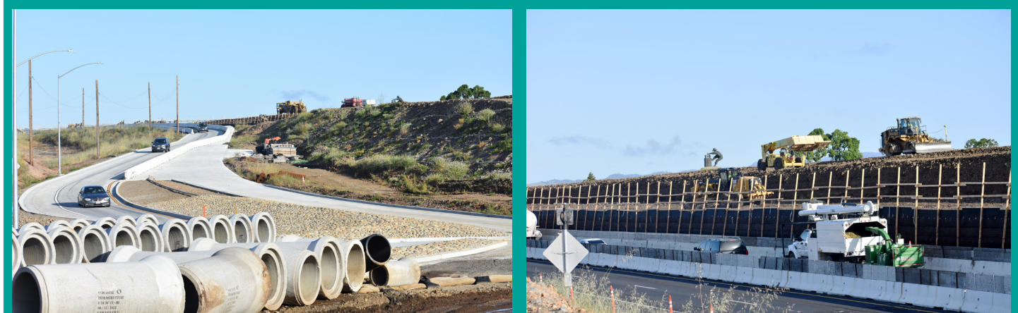
Current construction at Soscol Junction (May 2023)
