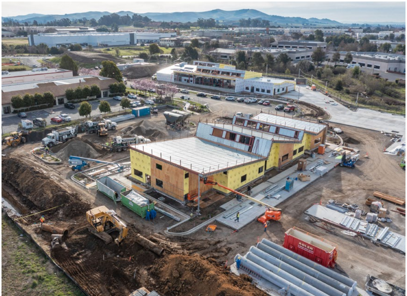
Current Construction, February 2023
