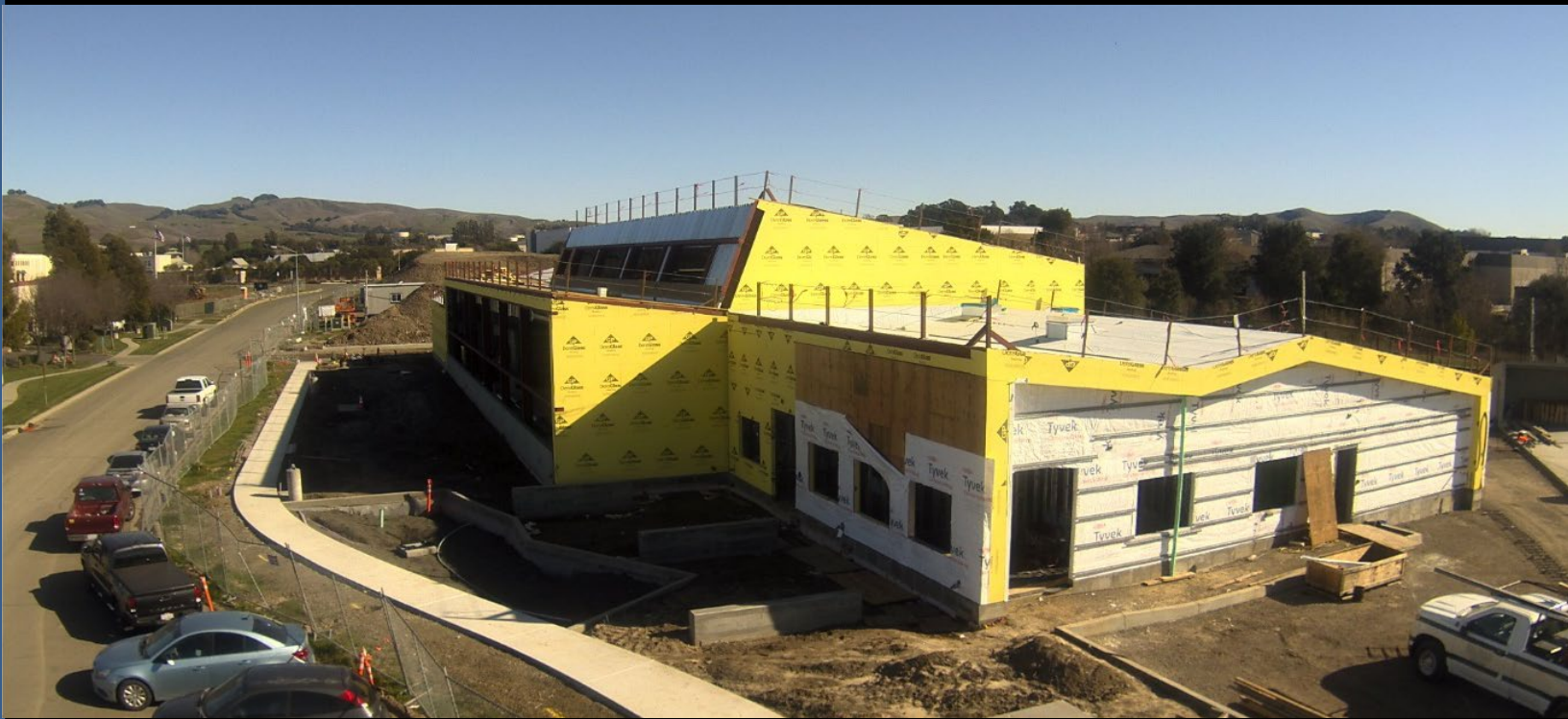
Vine Bus Maintenance Facility, February 2023
