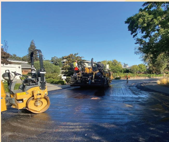
HERITAGE WAY (DURING CONSTRUCTION)
