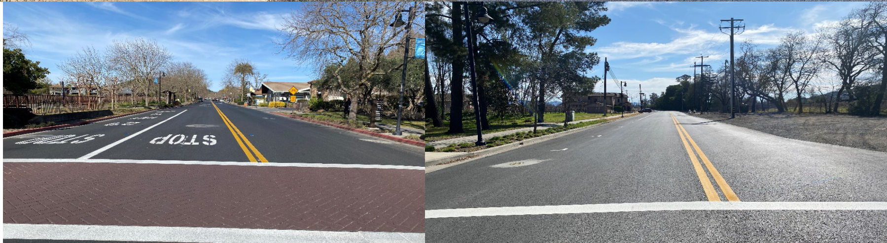
Washington Street South Rehab
